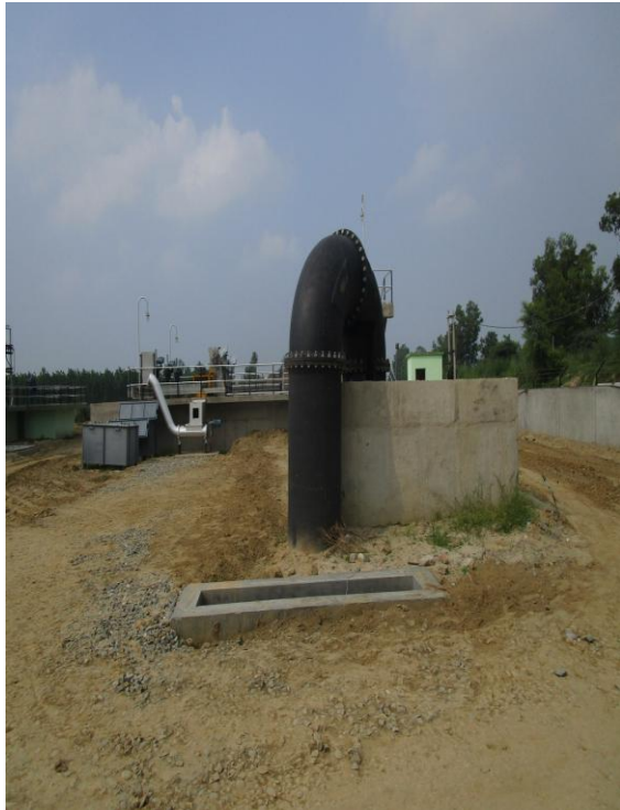
MAIN PUMPING STATION INLET:-
